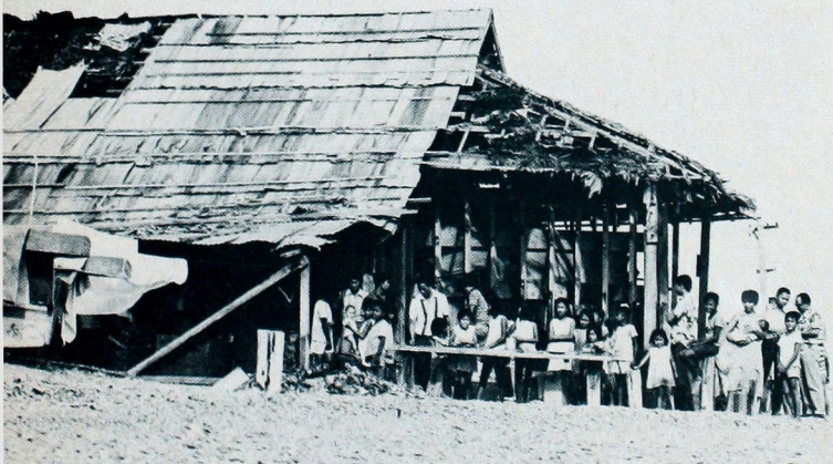
A warehouse evacuation center where 20 families live crowded into tiny cubicles with only rags dividing the spaces.
